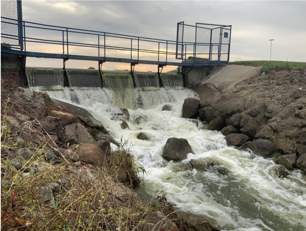
Lake Bel Air Dam – Hillsdale County
