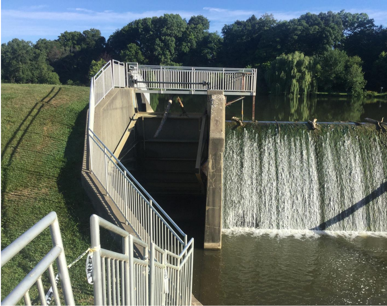
Saline River Dam– Washtenaw County
