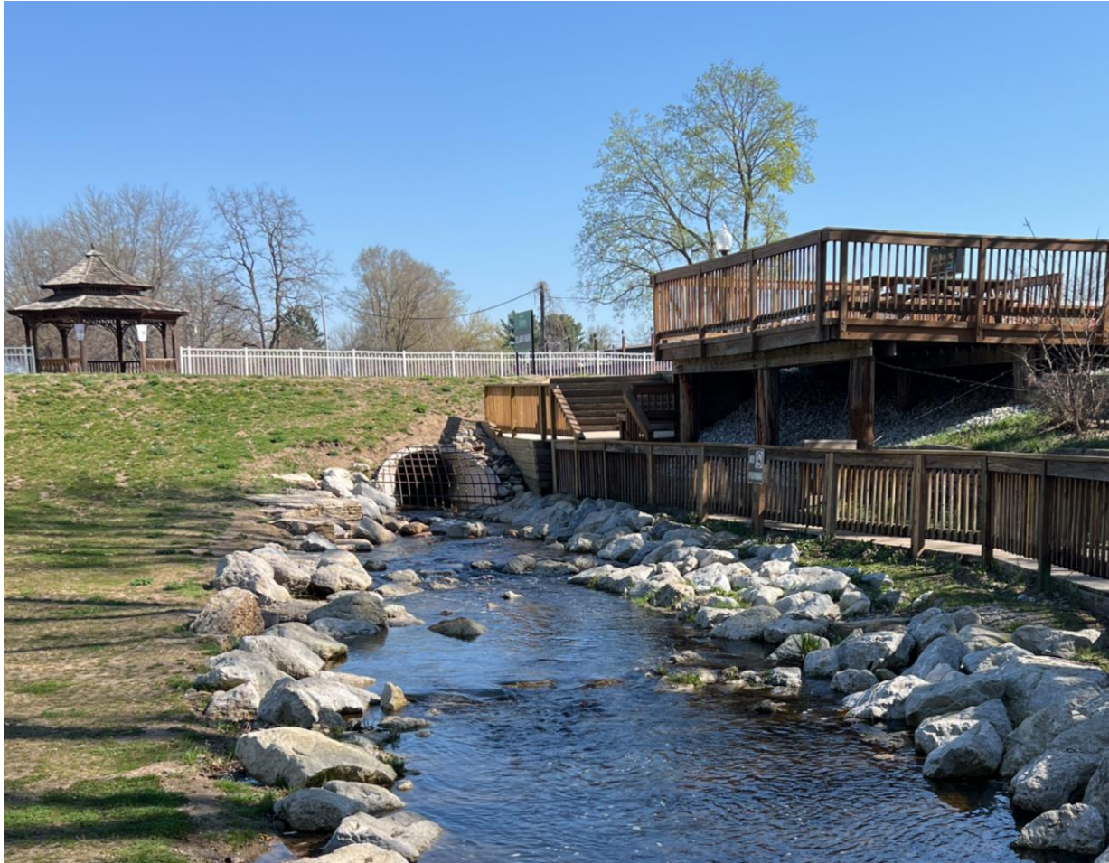
Sunset Lake Dam– Kalamazoo County
