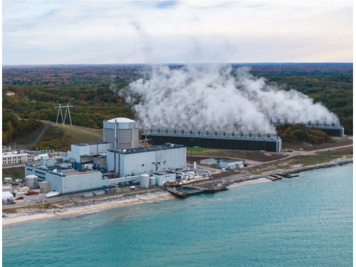
THE PALISADES NUCLEAR POWER PLANT IN VAN BUREN COUNTY HAS A NEW FUTURE THANKS TO EFFORTS BY LOCAL, STATE AND FEDERAL OFFICIALS. (PHOTO COURTESY OF HOLTEC INTERNATIONAL)
